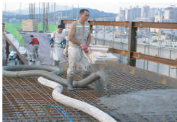
Bottom: Careful finishing of the KIM concrete rooftop slab.
