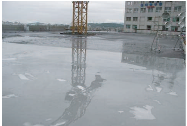
Above: The KIM concrete experienced less shrinkage and less cracking during the curing period.
