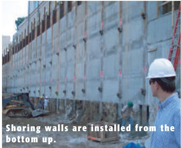
**Shoring walls are installed from the bottom up.**
