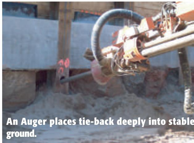
**An Auger places tie-back deeply into stable ground.**
